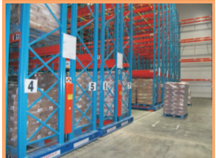
New mobile racked store at Farm Fresh, CT
